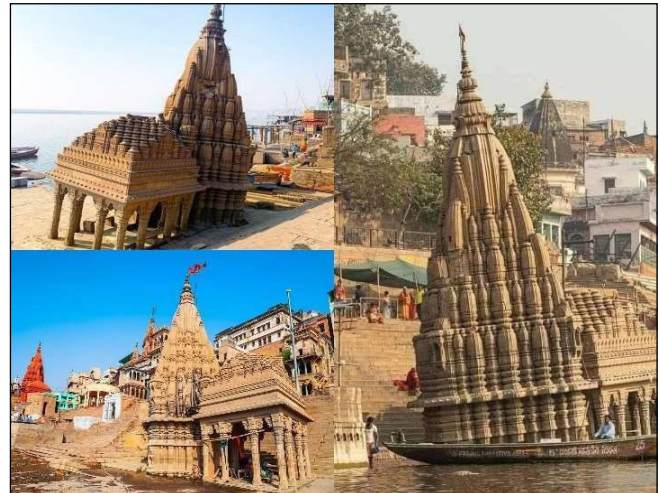
Figure 8. Ratneshwar Mahadev Temple Exterior View showing the tilted structure
