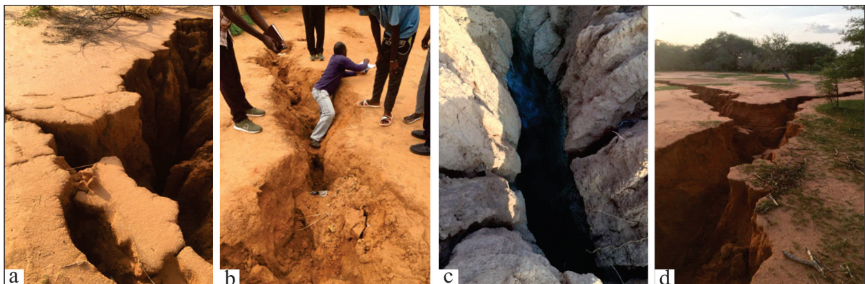
Figure 3. Cracks in many Parts displaying Collapses and their descent Down through the Crack Zone
